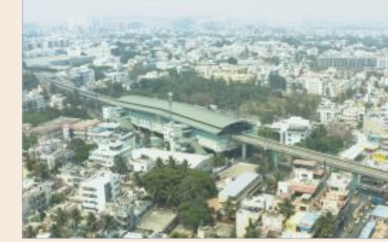
Yelachenahalli Metro Station - 100 Mtrs.
